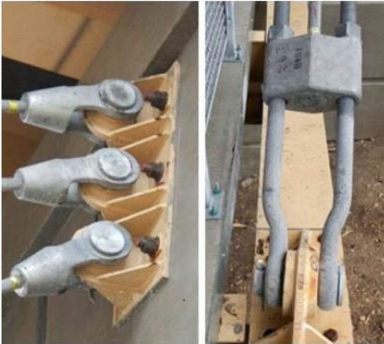
Upper and lower cable connection details
